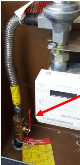
Your gas supply can also be turned off at the red handle isolation valve which is in the Brown Meter Unit on the outside wall
