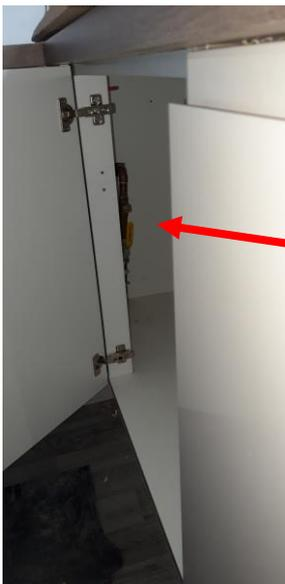
Your gas supply can also be turned off at the yellow handle isolation valve which is in the kitchen cupboard underneath the sink
