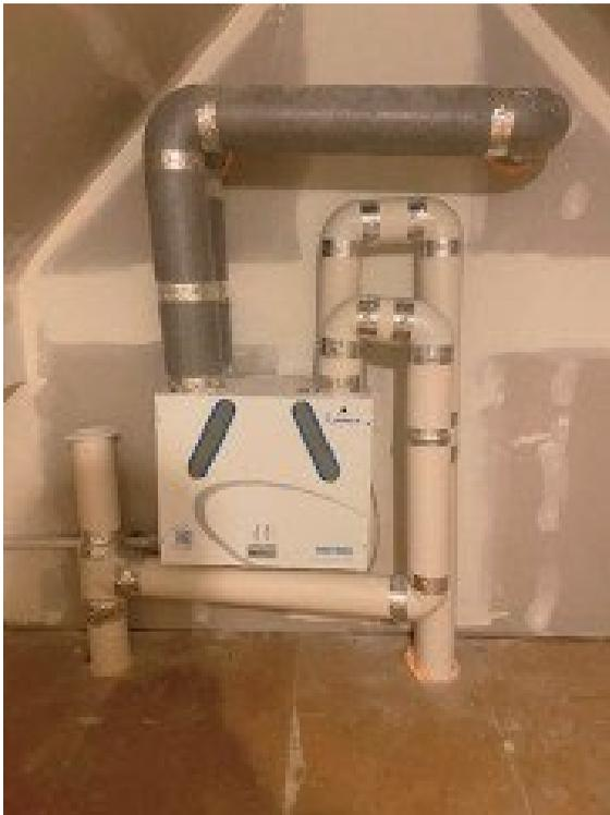
This is a typical example of the MVHR system installed at Gwynfaen. The system can keep up to 95% of heat that's normally lost through open windows, trickle vents and extractor fans, allowing you to make energy savings. It's like recycling warm air from one part of your house to another.
