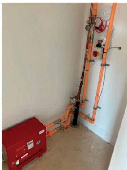
If you ever need to turn off your water, the stopcock, it is located in the cupboard underneath the stairs adjacent to the sprinkler pump. A typical example is shown in the photo.
